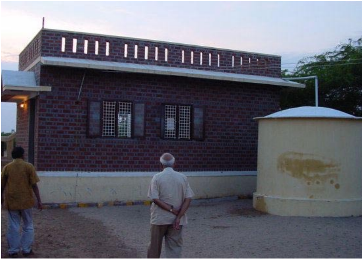
A typical center - with rain water harvesting !
